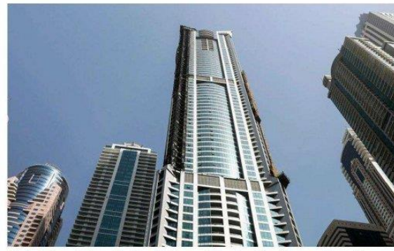
(b) The Torch Building (Dubai) after the fire
