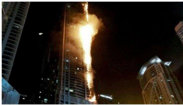
(a) The Torch Building (Dubai) during the fire
