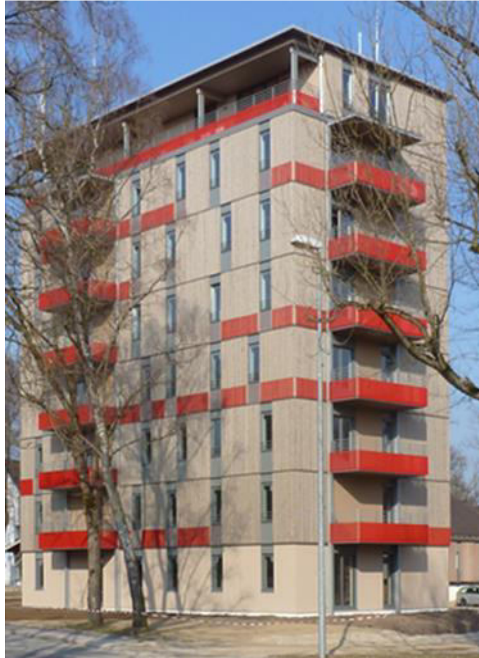
H8, Bad Aibling, City of Wood, B&O Schankulla Architekten, Bj. 2011
